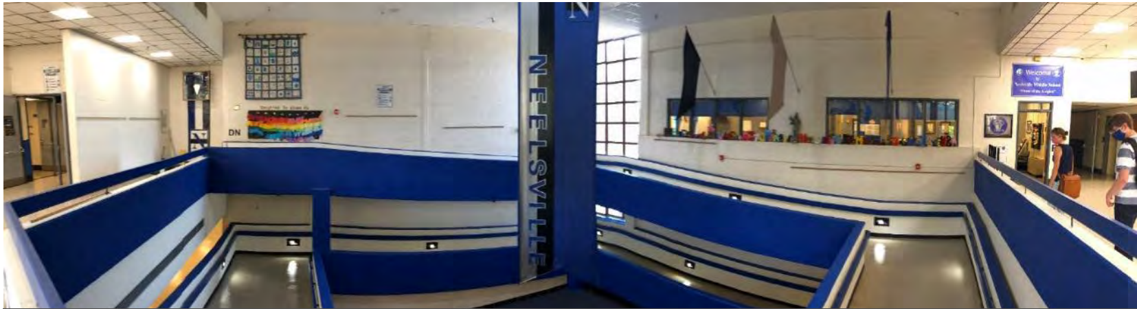
INSUFFICIENT SECURITY; INACCESSIBLE RAMP; LACK OF ELEVATOR
