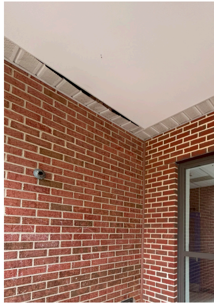
Soffit Opening
