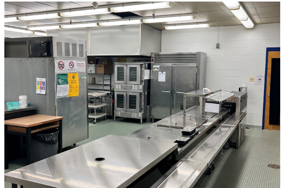
Existing kitchen area
