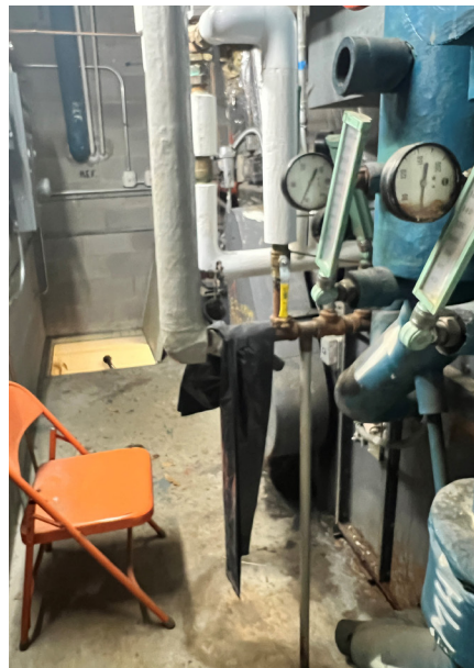
Existing air handling unit for multipurpose room
