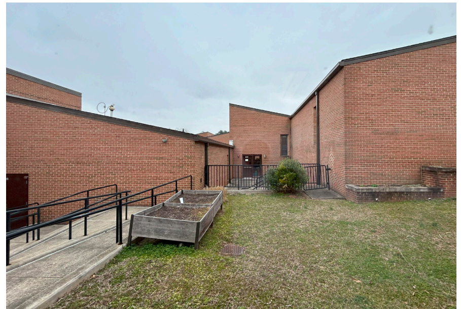
Large Existing Courtyard
