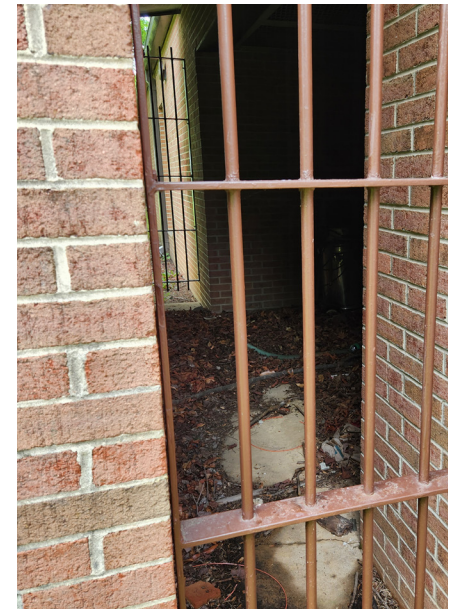
Enclosed Exterior Space on South Facade
