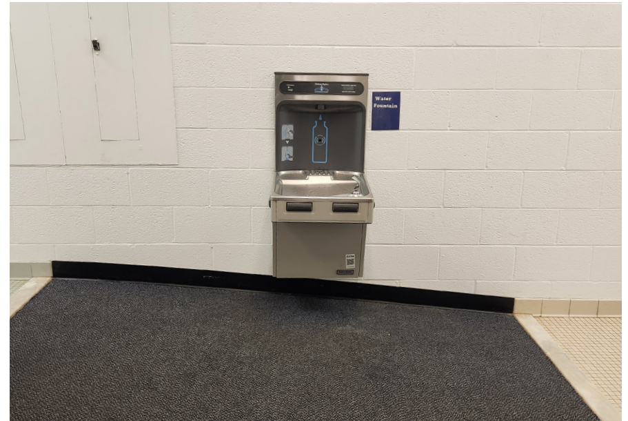
Ramp at Restroom Entry
