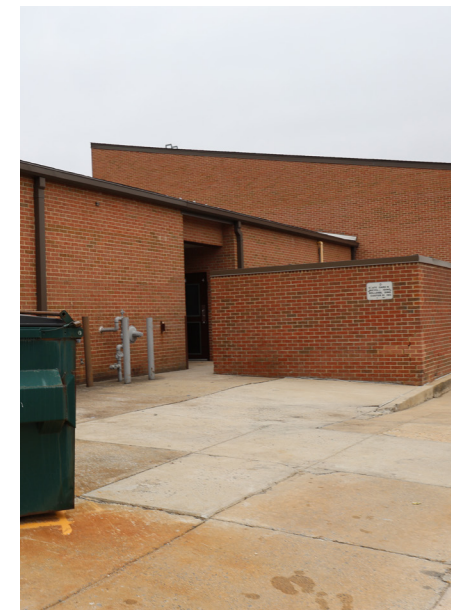
Service Area - Open Enclosure
