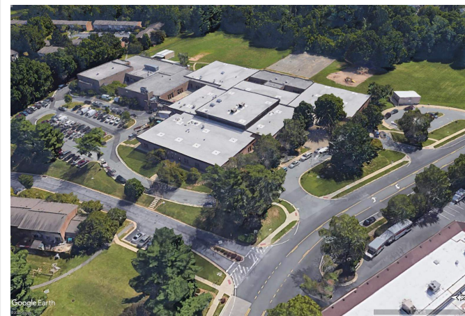
View from West
