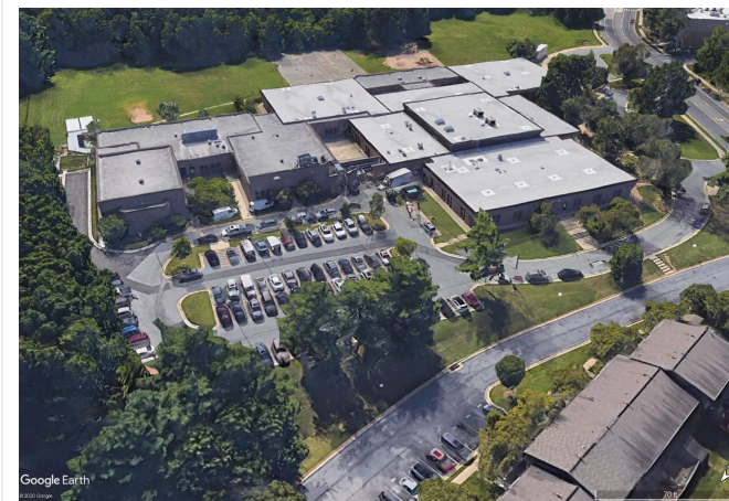
View from North
