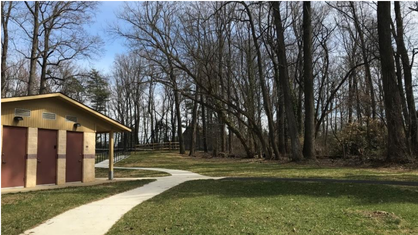
STRATTON LOCAL PARK-site photo
