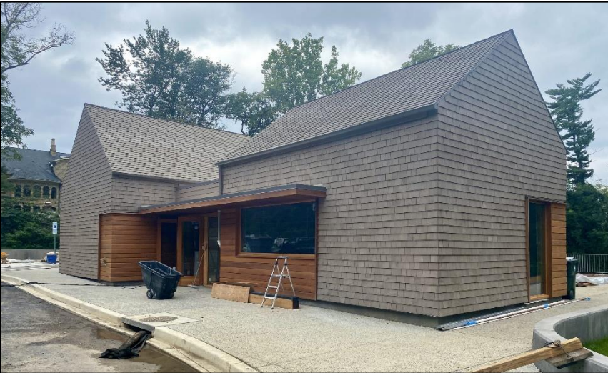
The Josiah Henson Park Visitor Center/Museum nears completion.
